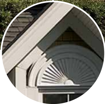
Sheets routed into sunburst window header with heat formed Back Band.
