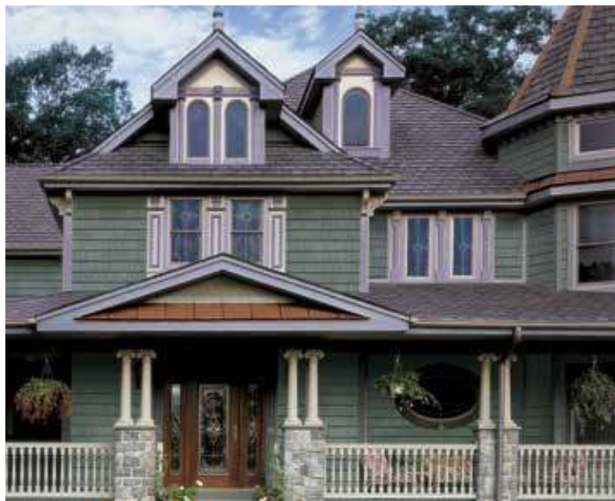
Custom-painted Restoration Millwork
